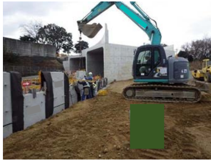
壁面材組立て
