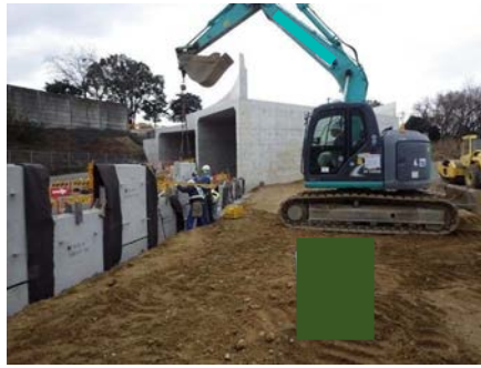
壁面材組立て
