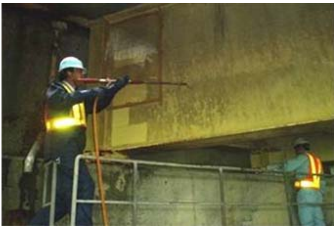
桁端部塩分洗浄状況
