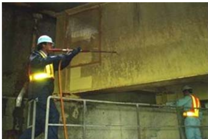
桁端部塩分洗浄状況
