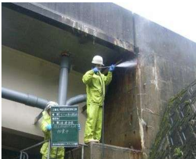
桁端部塩分洗浄状況
