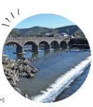
耶馬溪橋 Yamabiki bridge
