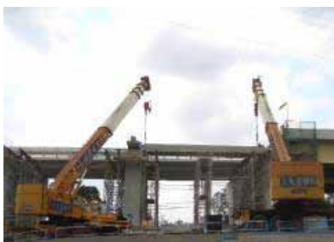
(橋梁修繕の実施例)
